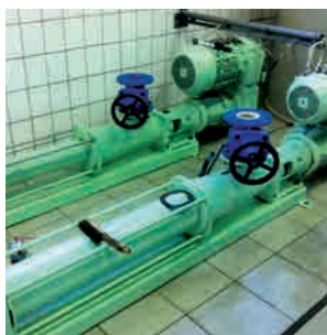
Conveyance of thin slurry: KL50S progressing cavity pump
