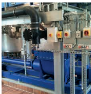
Conveyance of sludge from decanter to silo: KL65RÜ80.4 ESP with fill level monitoring
